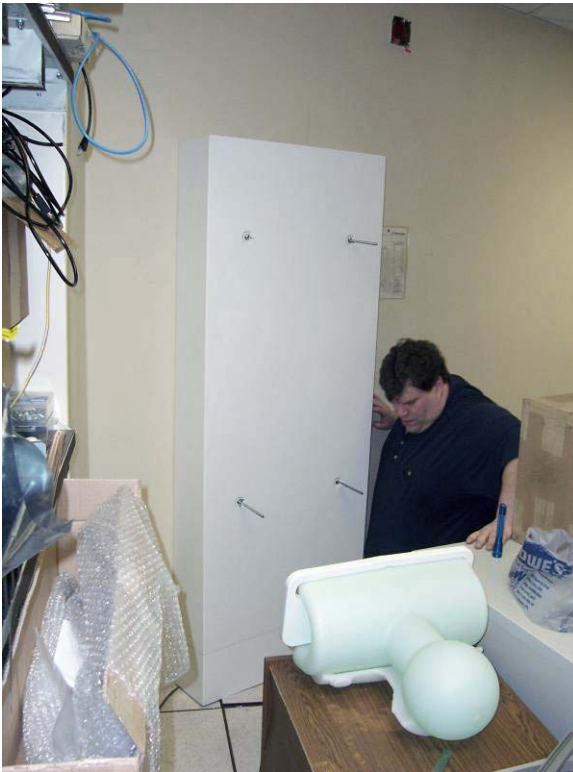
Engineer examining removed shield panel in equipment room
