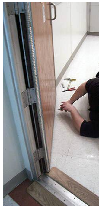
Engineer replacing damaged fingerstock
